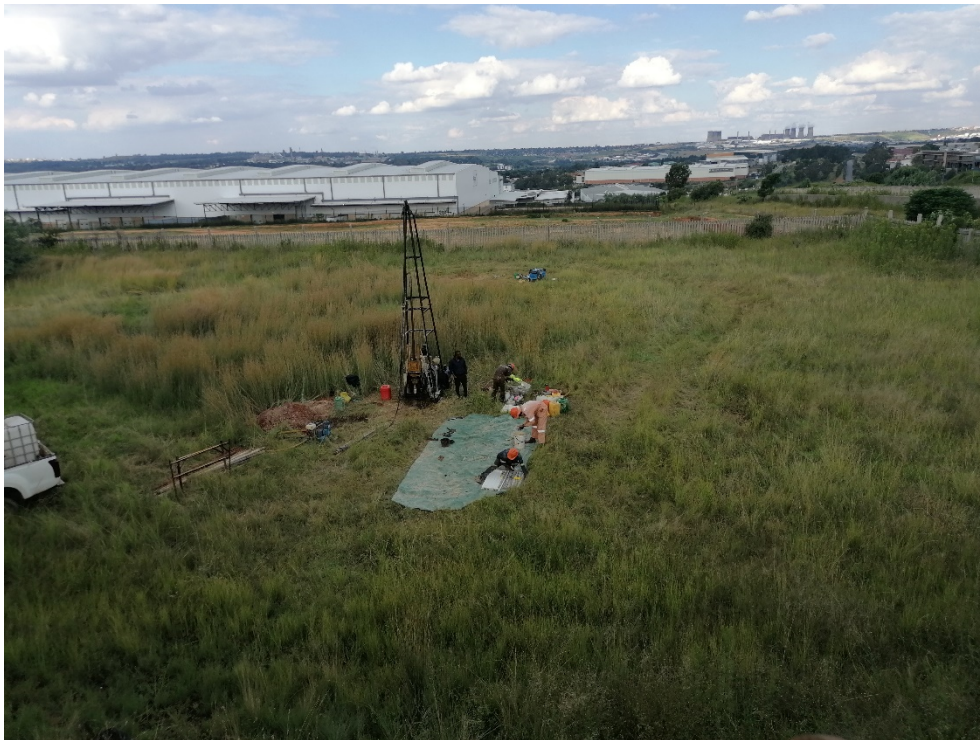
Plate 2: View towards the east from the existing reservoir, note drilling of BH02
