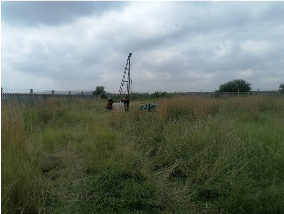
Plate 1: View towards the south, note drilling of BH01
