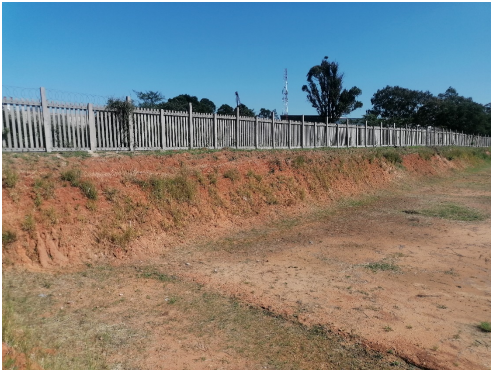
Plate 4: View towards the west from adjacent property, note deep excavations
